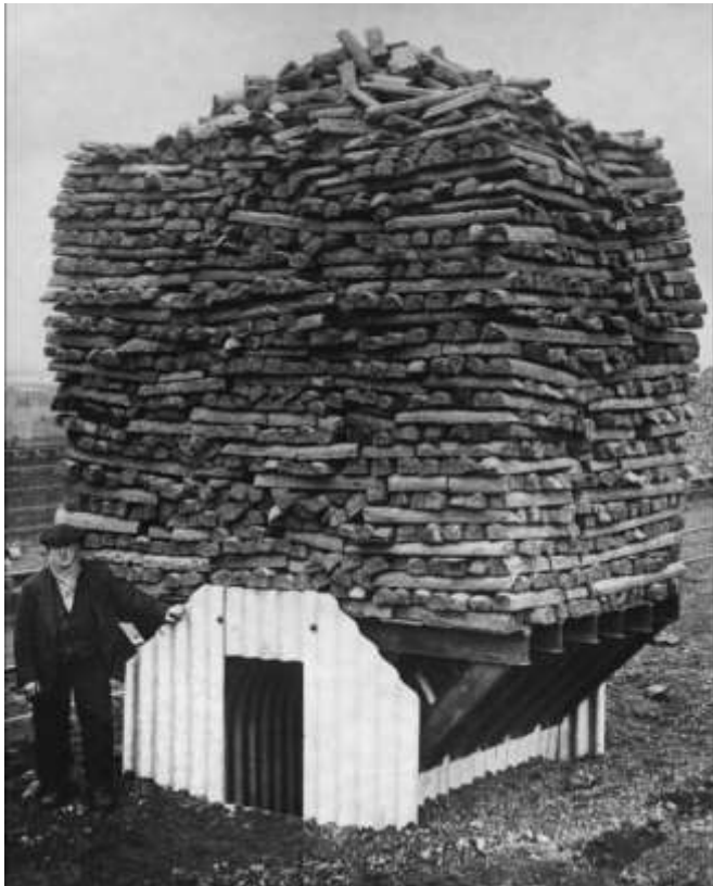
This image taken in 1939, somewhere in Wales was a test rig to see how much stain could be put on the roof 75 tons of Pig Iron and the structure remained stable
